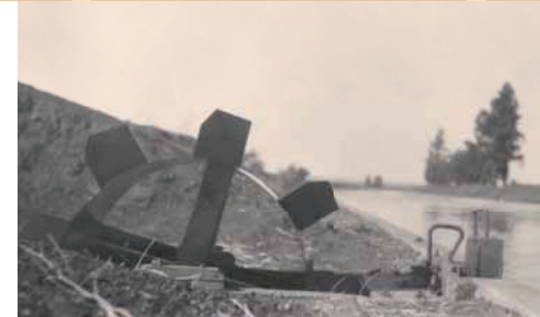
Dethridge wheel on a farm in Lake Wyangan, 1922. GRIFFITH CITY LIBRARY
